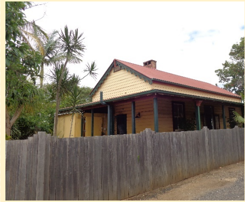
Side fence left to weather off
