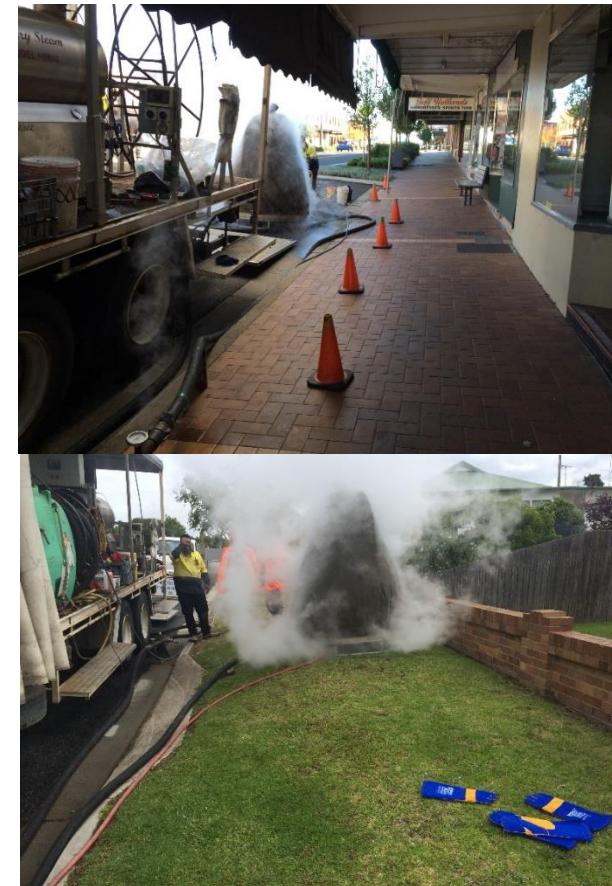
Sewer re-lining (photos: Melissa Blum)
