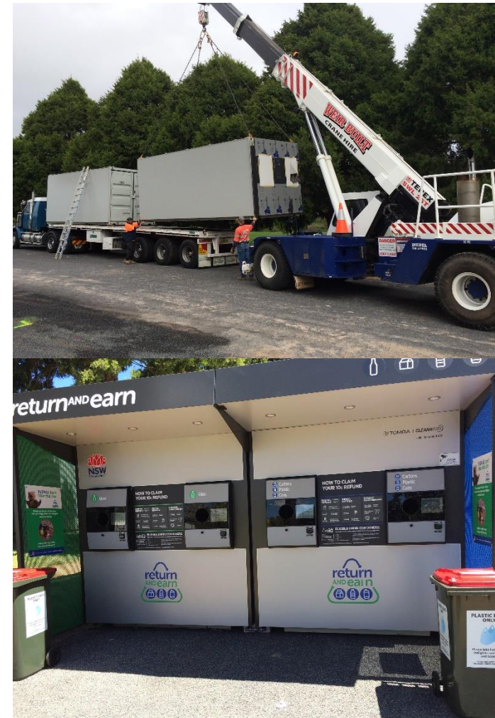
Installation of Container Deposit Scheme Automatic Reverse Vending Machines (photos: Melissa Blum)
