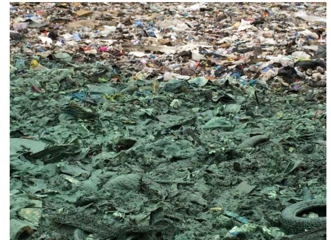
Posi-shell trial for alternative daily cover for waste landfill (photo: Melissa Blum)
