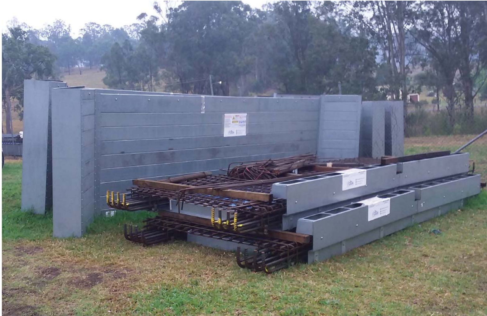
InQuik Bridge – to the right is the deck, to the left is abutments and wingwalls. Geotechnical investigations are completed at each site to determine a suitable footing.
