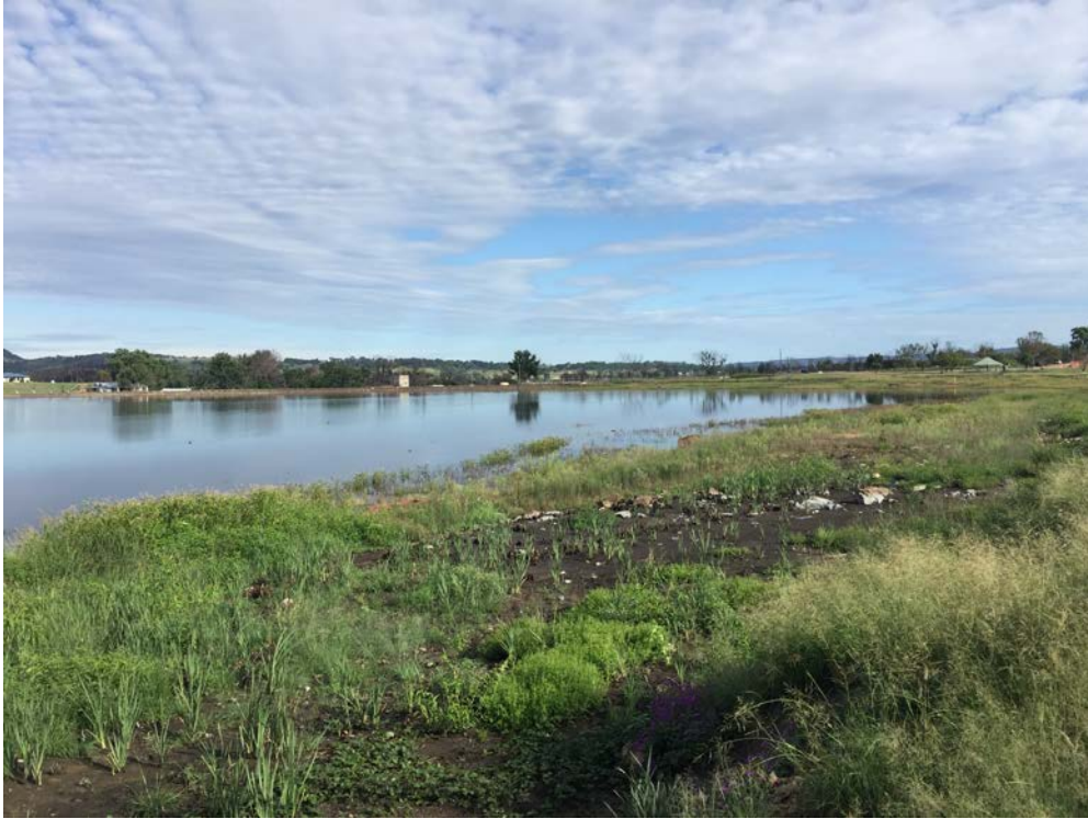
Tenterfield Dam at 60% capacity – Looking north towards the wall
