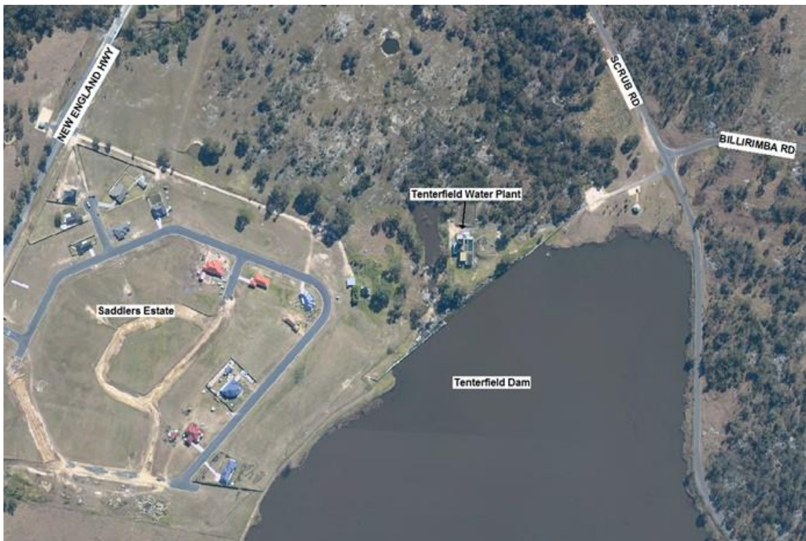
Figure 2 Tenterfield Water Supply Dam & Water Treatment Plant
