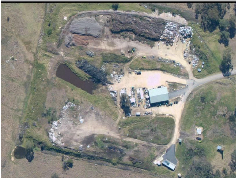
Figure 4-3 Tenterfield Waste Transfer Station
