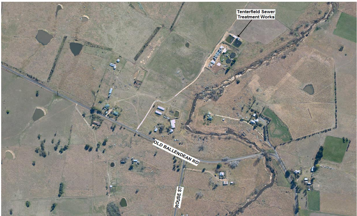
Figure 11 Tenterfield Sewerage Treatment Plant
