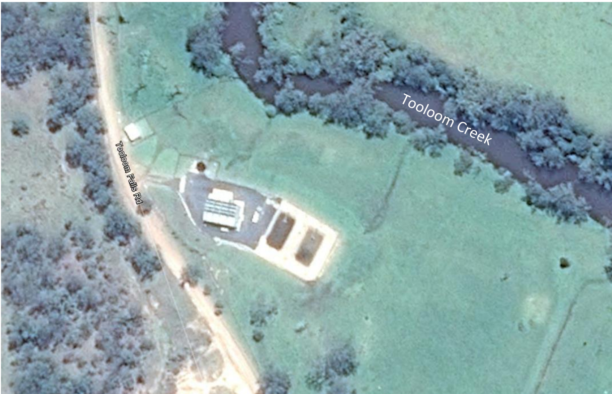
Figure 5 Urbenville Water Treatment Plant
