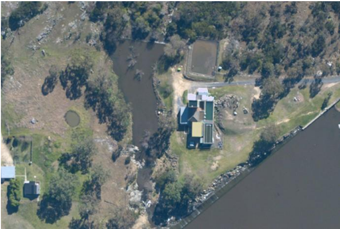
Figure 3 Tenterfield Water Treatment Plant
