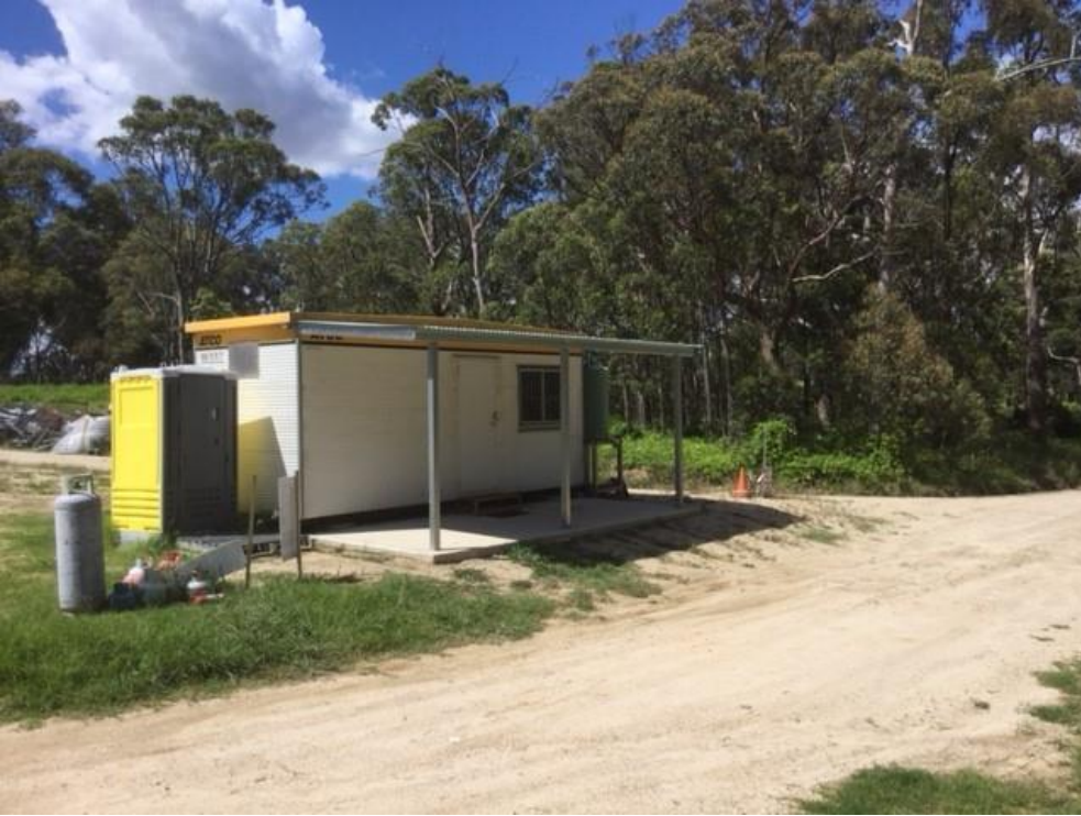
Figure 4-4 Liston Waste Transfer Station
