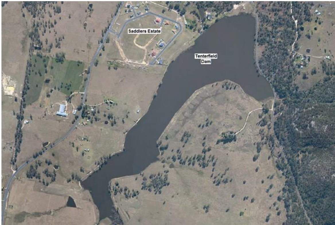
Figure 1 Tenterfield Water Supply Dam
