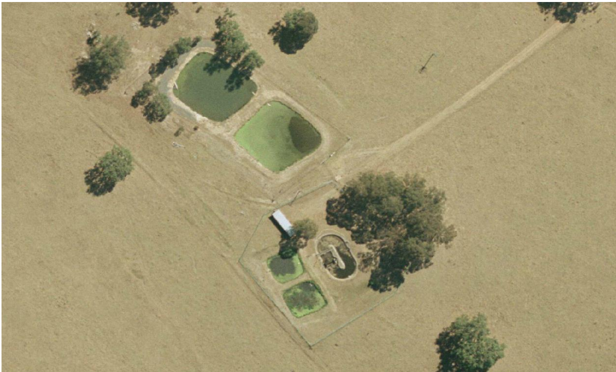
Figure 15 Urbenville Sewerage Treatment Plant
