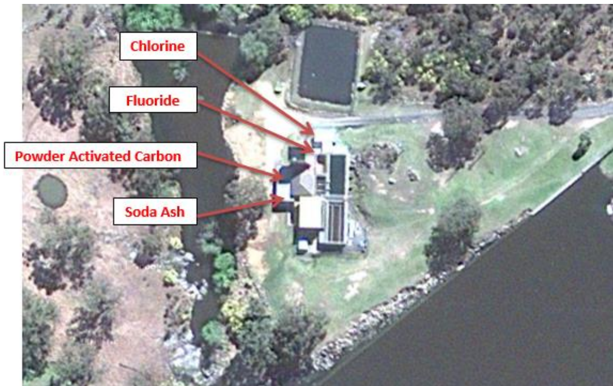
Figure 4 Tenterfield Water Treatment Plant – Location of Chemical Storages
