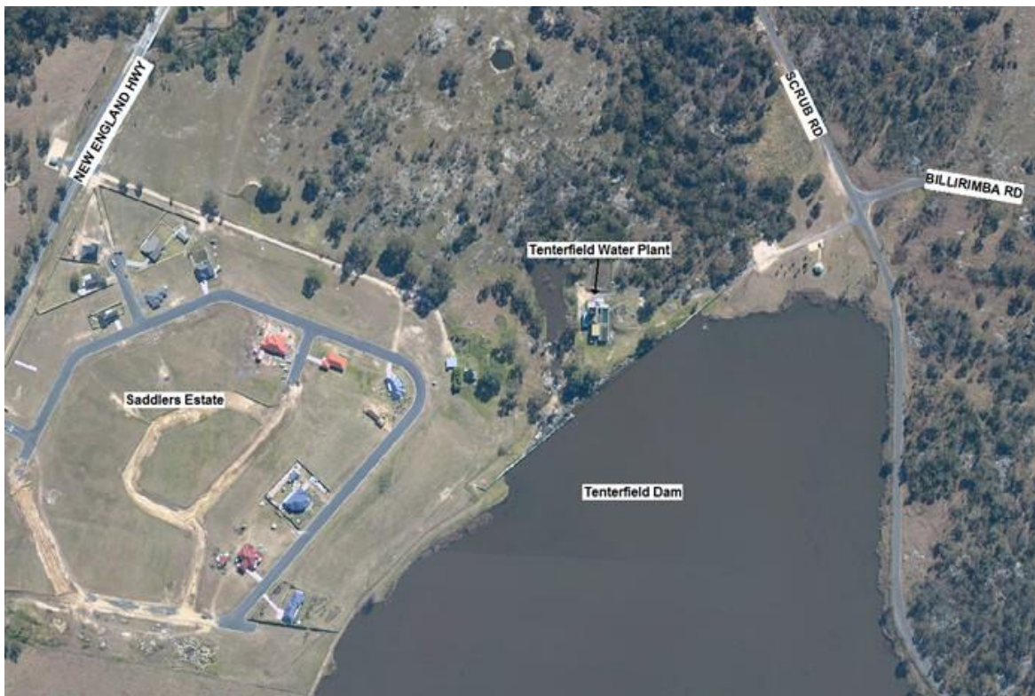
Figure 2.2 Tenterfield Water Supply Dam & Water Treatment Plant
