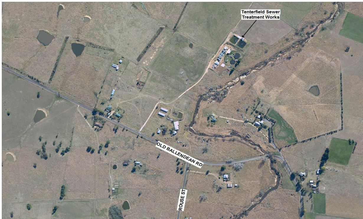
Figure 3-3 Tenterfield Sewerage Treatment Plant
