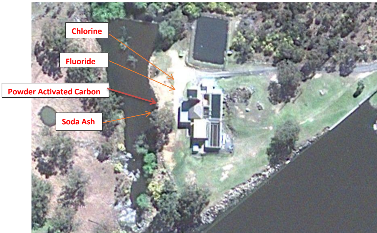
Figure 2.4 Tenterfield Water Treatment Plant - Location of Chemical Storages
