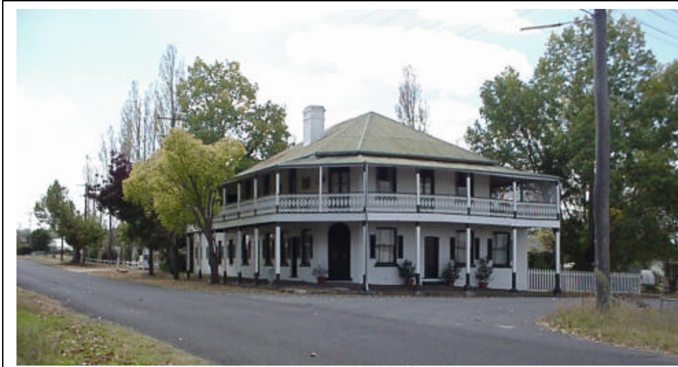
Tenterfield Lodge in Railway Avenue is the town's last surviving intact example of over-the-footpath verandahs that once dominated the central business area in Rouse Street.
