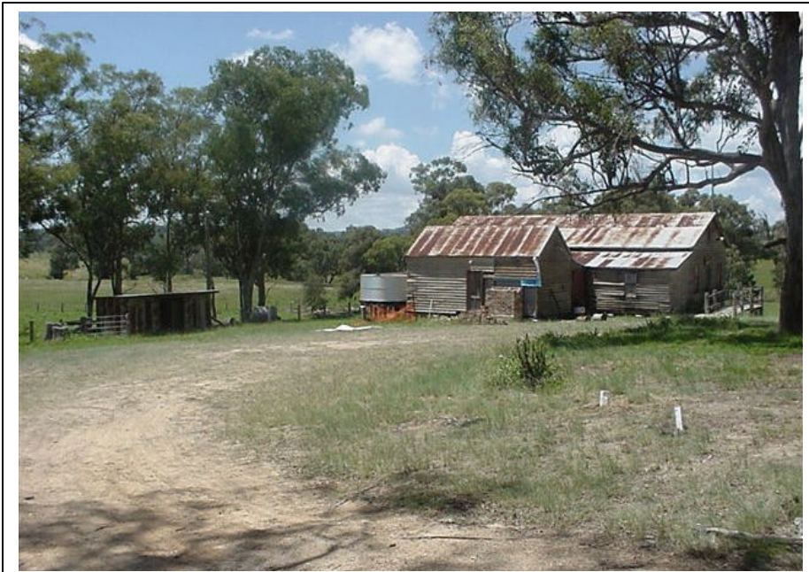
Steinbrook Hall ... one of 58 community nominations recorded on the non-statutory Local Heritage Register (2 of 2).
