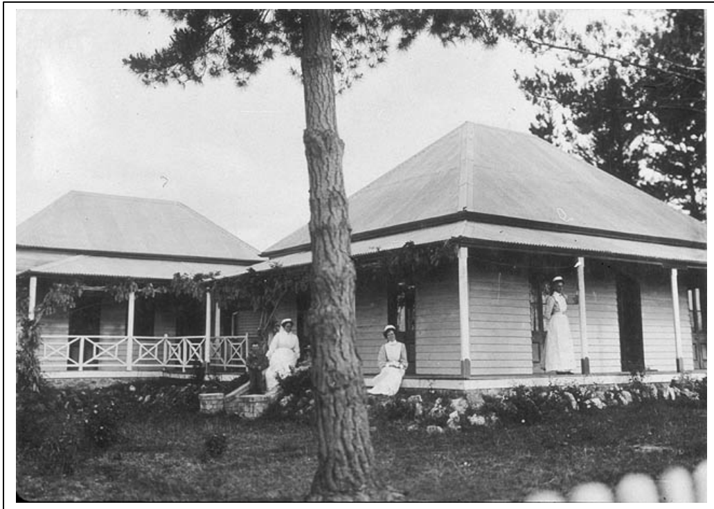
Torquay Hospital (1907-1940) at 84 Bulwer Street, now a private residence . See page 2.
