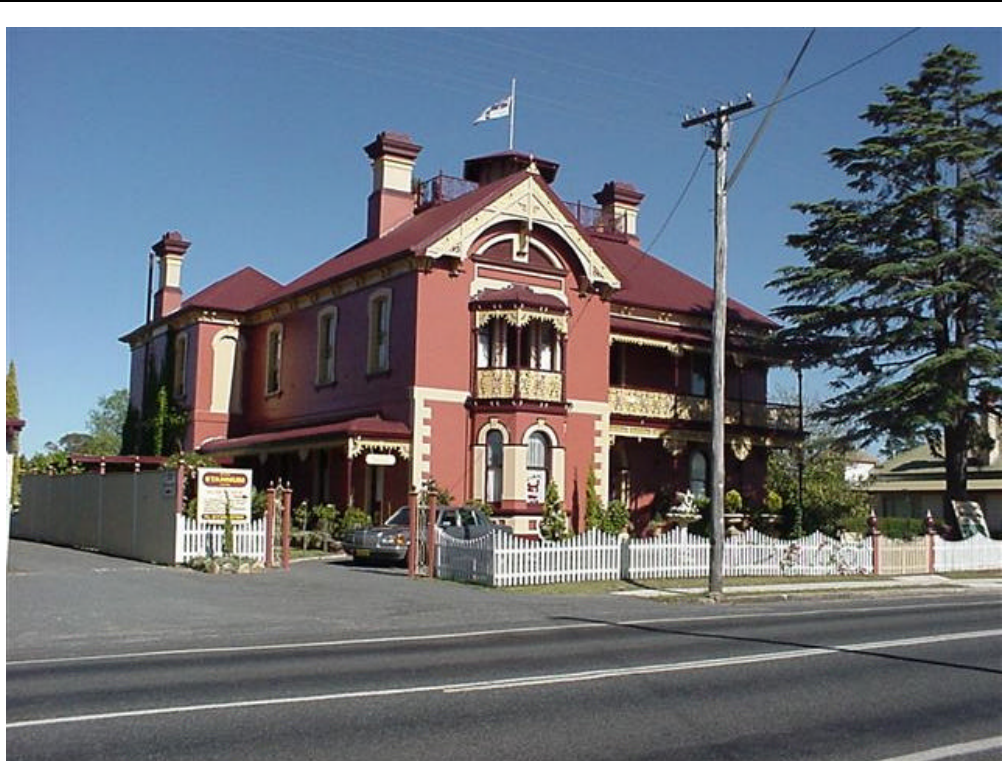
Stannum house on the entrance to Tenterfield's central business area is a rare Victorian Italianate home of triple brick with lavish cedar appointments and nine fireplaces of Italian marble. It was built by successful mining operator John Reid in the 1880's as a family home with a commanding view of the town from its tower.
