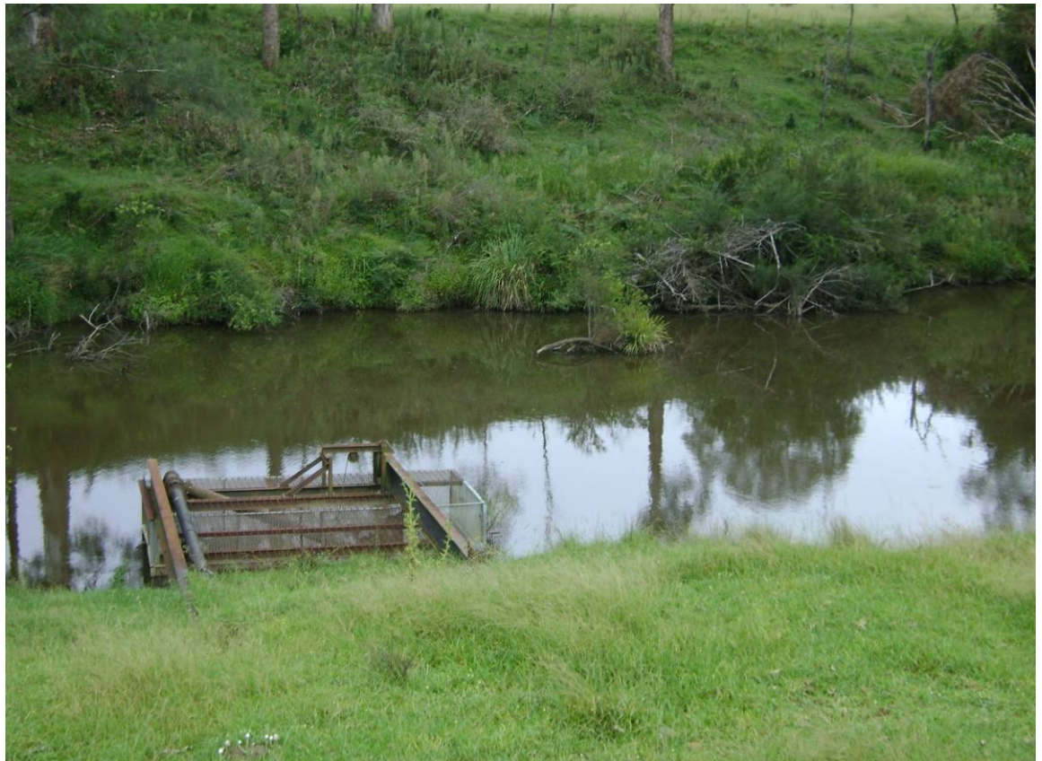
Figure 3-10: Tooloom Creek extraction structure
