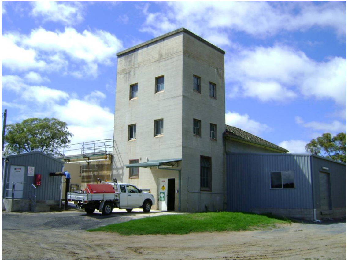
Figure 3-11: Tenterfield Water Treatment Plant
