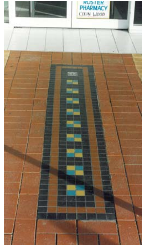
Town Centre Footpath Treatment 1 : Turn over existing pavers, relay on a better base, build in colour tile carpets on concrete base at key points
