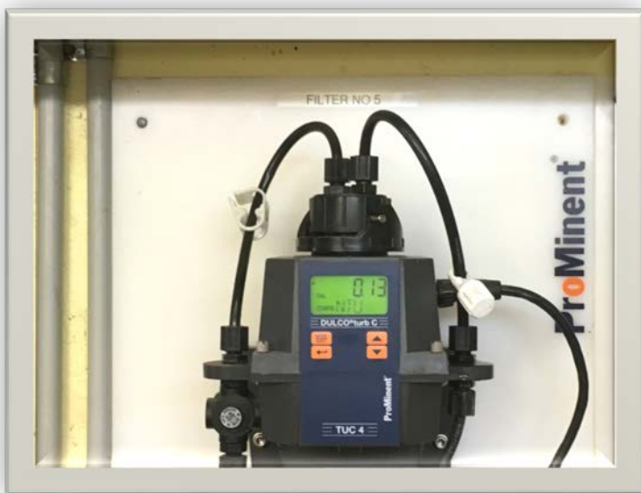
Figure 18, 19 & 20 New on-line turbidity meters installed December 2019.
