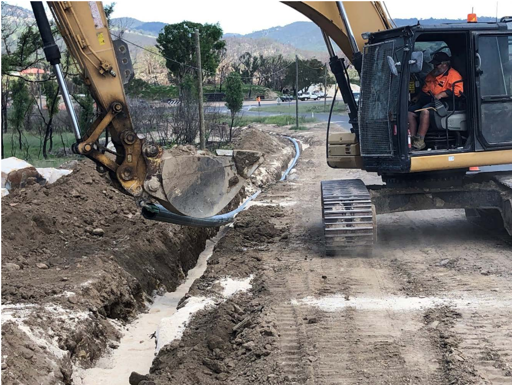
Laying pipe for bores on Billirimba Road
