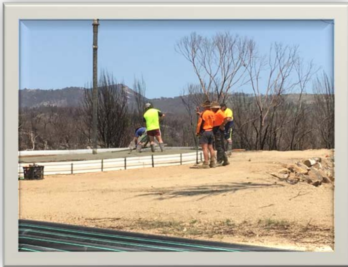
Figure 21, 22 & 23 Installation of new pad for holding tank at dam December 2019.
