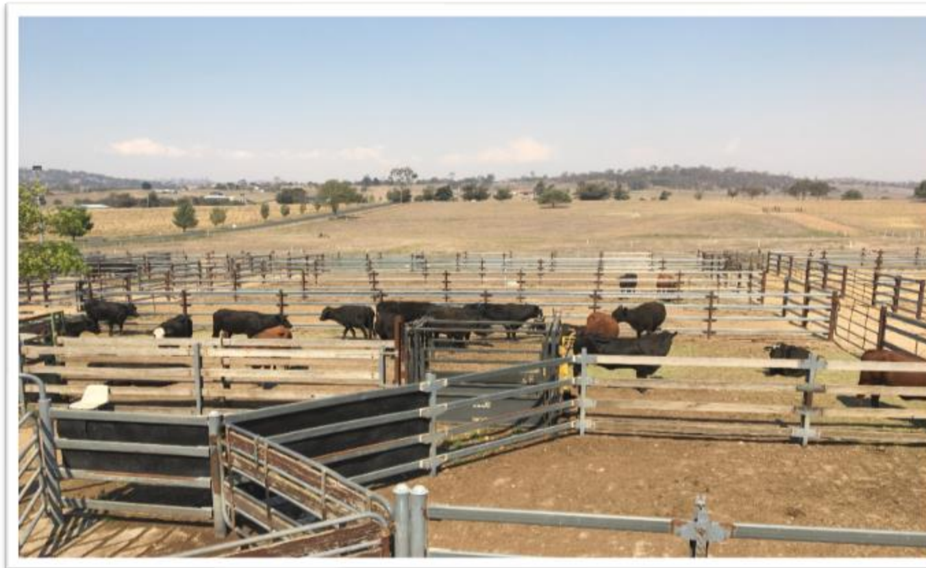
New replacement steel rails to holding pens
