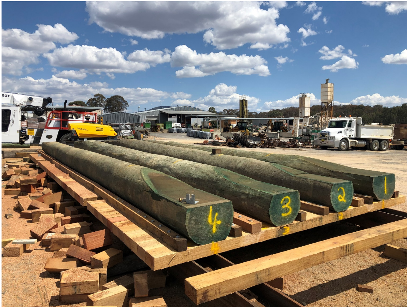
Silent Grove Rd Bridge superstructure constructed in the depot for more efficient costing
