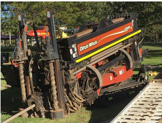
Underboring equipment at work near Tenterfield Creek
