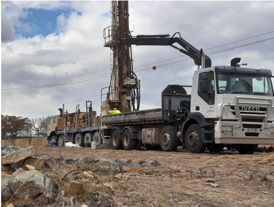
Drilling for Water
