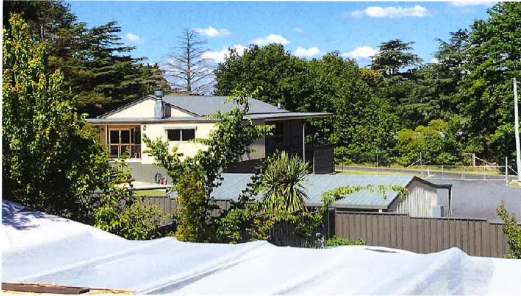
Photo 5: View from rear of 53 George Street
