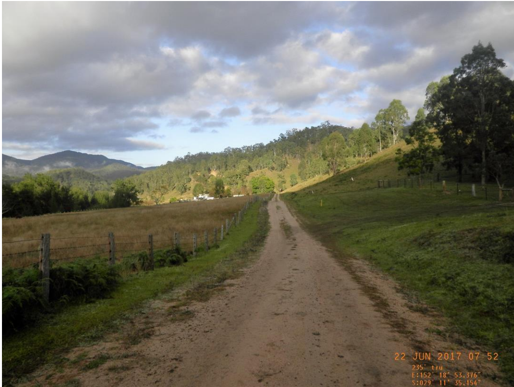
Photo #1 – Facing towards Billirimba Road showing sight distance of 200m
