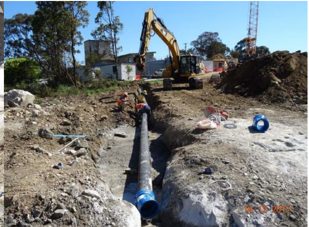
Installation of the 250 dia Outlet pipework
