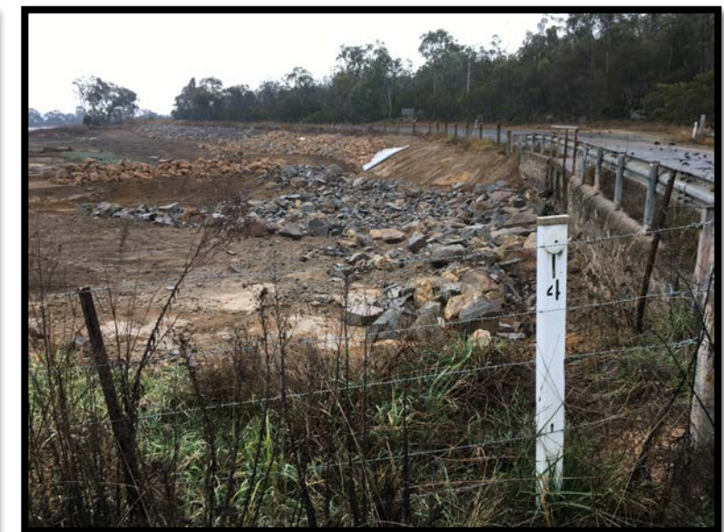
Figure 2 and 3 Tenterfield Dam Bank reinforcement/restabilisation Eastern inlet - July 2019
