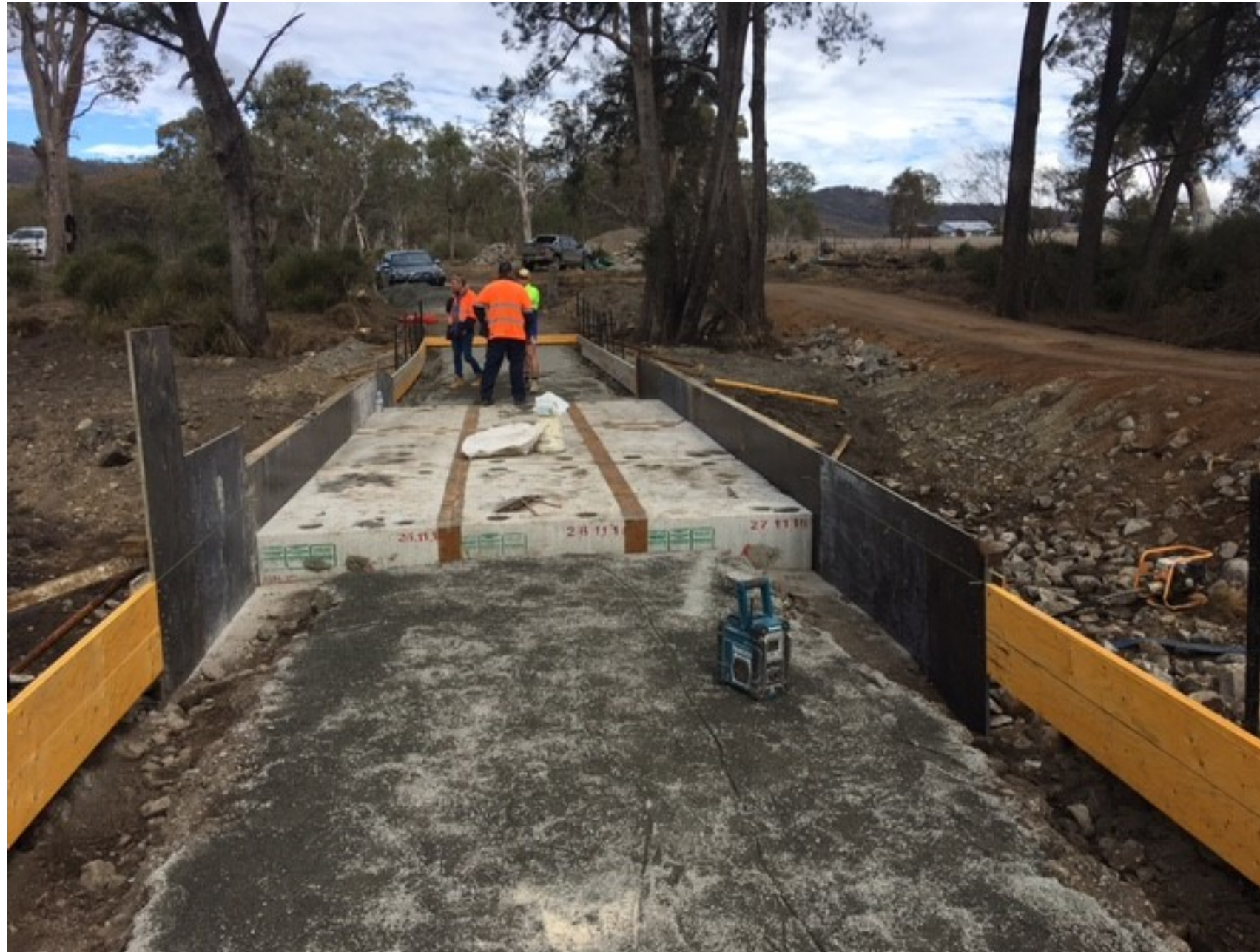
Sawyers Gully Rd – preparation to install mesh and pour the top deck 09-07-2019
