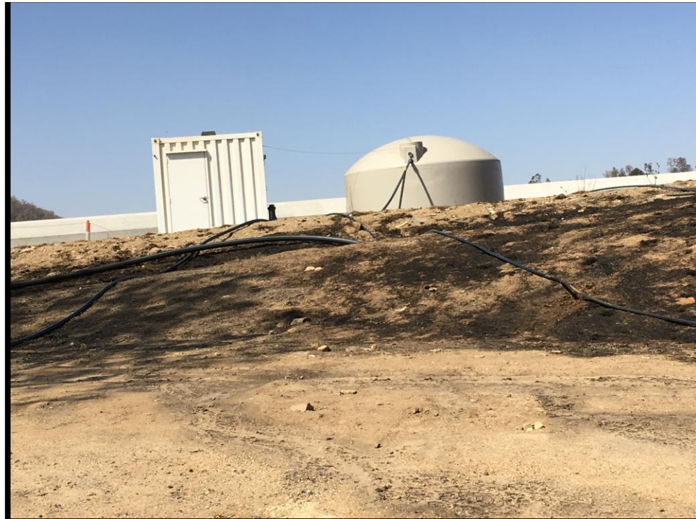
Figure 6 RO/Desalination Plant survived with no damage; however feed pipes damaged September 2019
