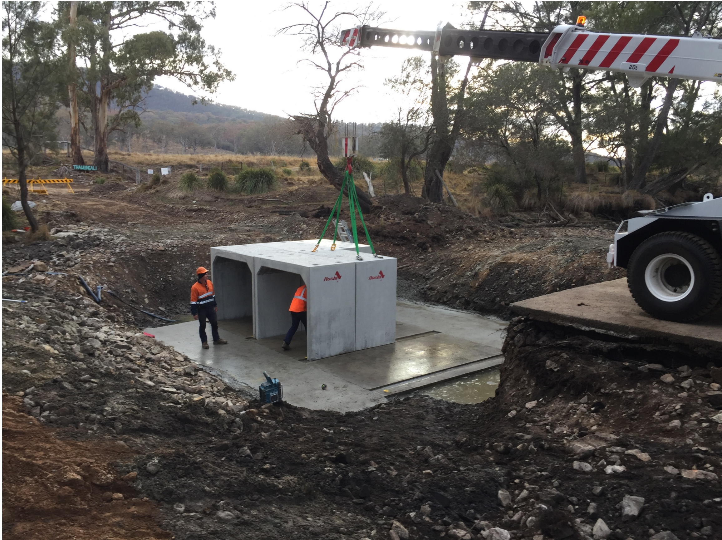
Placing of culverts at Sawyers Gully Rd
