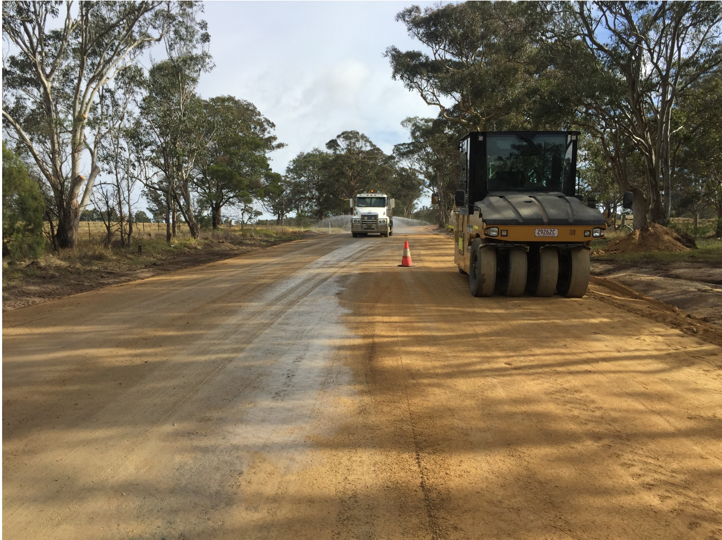
Amosfield Rd – Full reconstruction of subbase.
