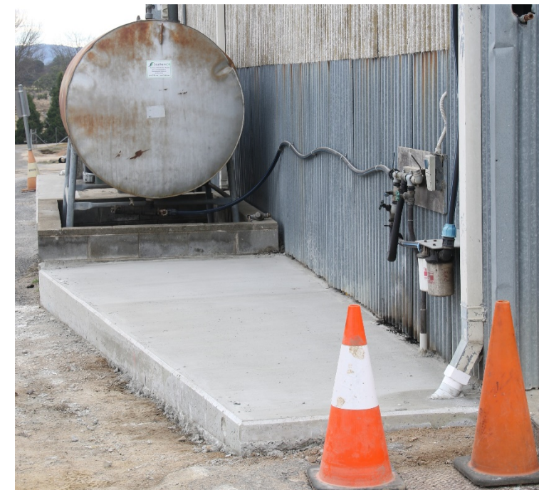
Concrete footing for new bulk oil storage are
