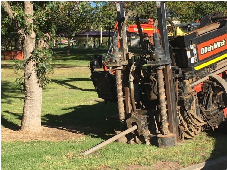
Figure 6 Under- boring machine at Link Street
