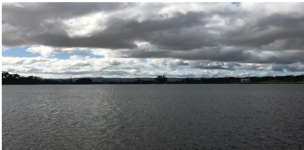
Figure 3: Tenterfield Dam 7 May 2020
