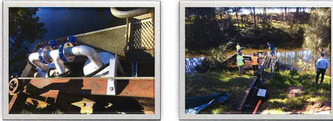
Figure 4 & 5 Replacement submersibles and Onsite inspection
