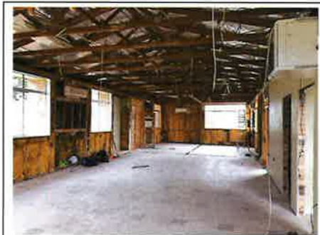
Riley Street Depot - Demolition
