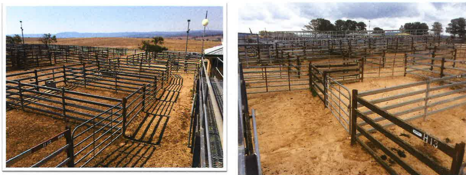
New replacement steel rails to holding pens before and after photos.
