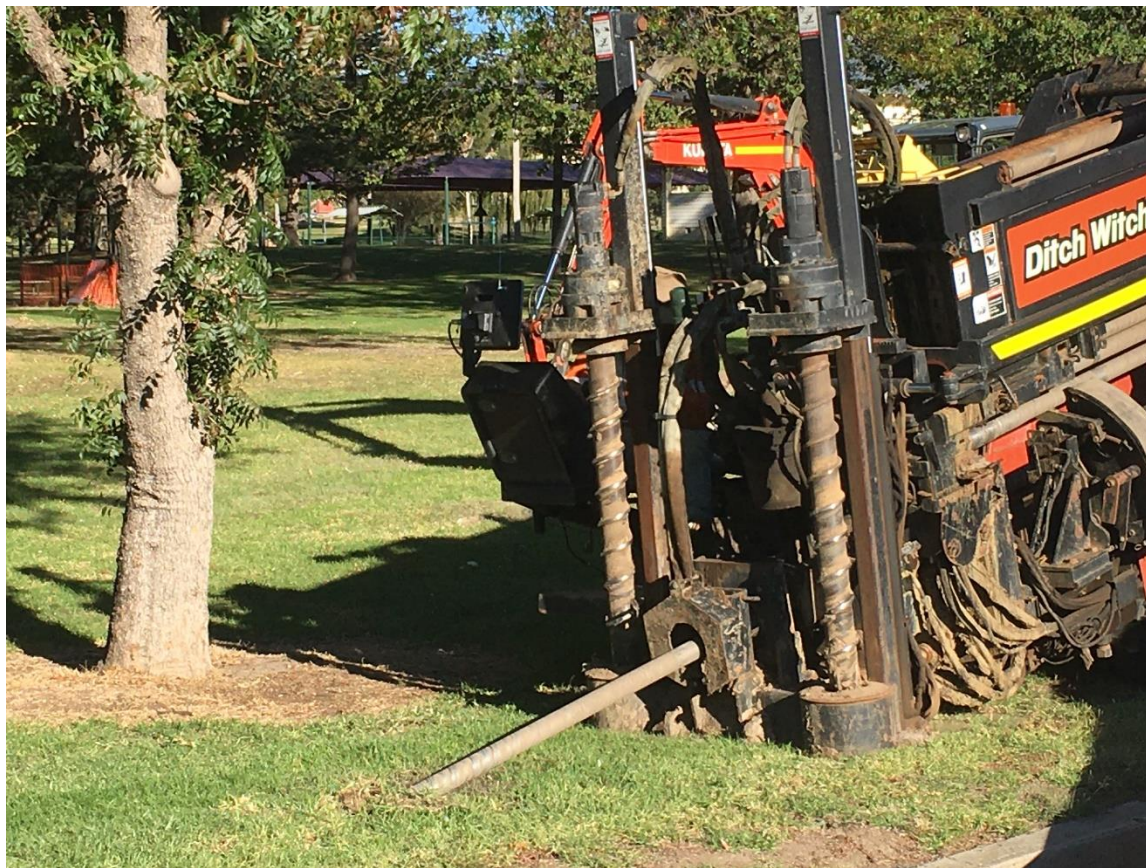
Figure 6 Under- boring machine at Link Street
