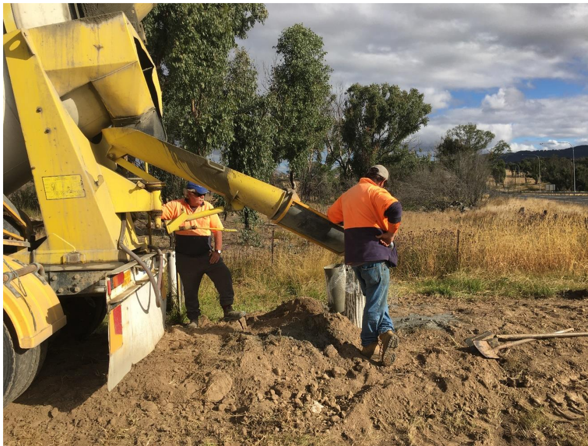
Figure 7 Grouting the pipes on the New England Highway under bore
