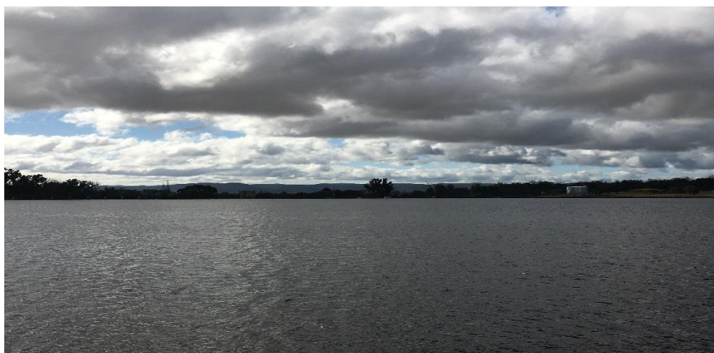
Figure 3: Tenterfield Dam 7 May 2020
