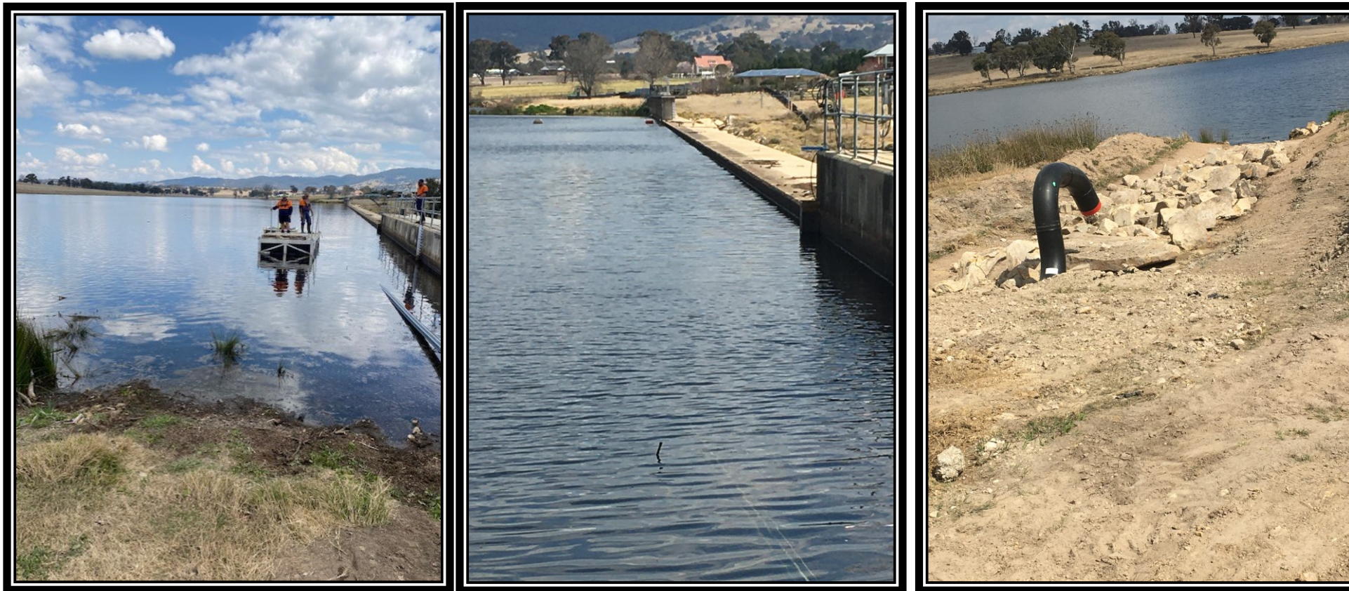
Figure 1, 2 and 3 Aerator pipe installation with pontoon barge, sunken aeration line; and, Bore waterfall.
