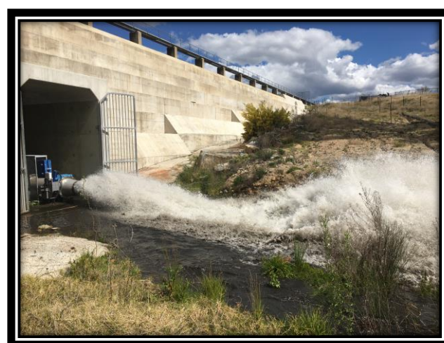
Figure 7, Example of Gate Valve Opening in September 2020
