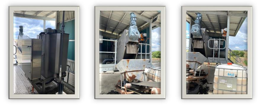
Figure 1, 2 and 3 Tenterfield new Dehydrator (Sludge press) in operation.
