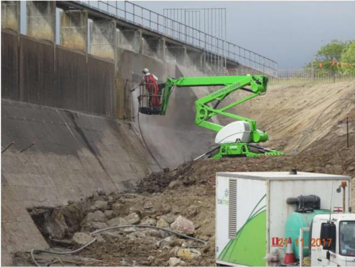
Hydro-Cutting Dam Wall Concrete
