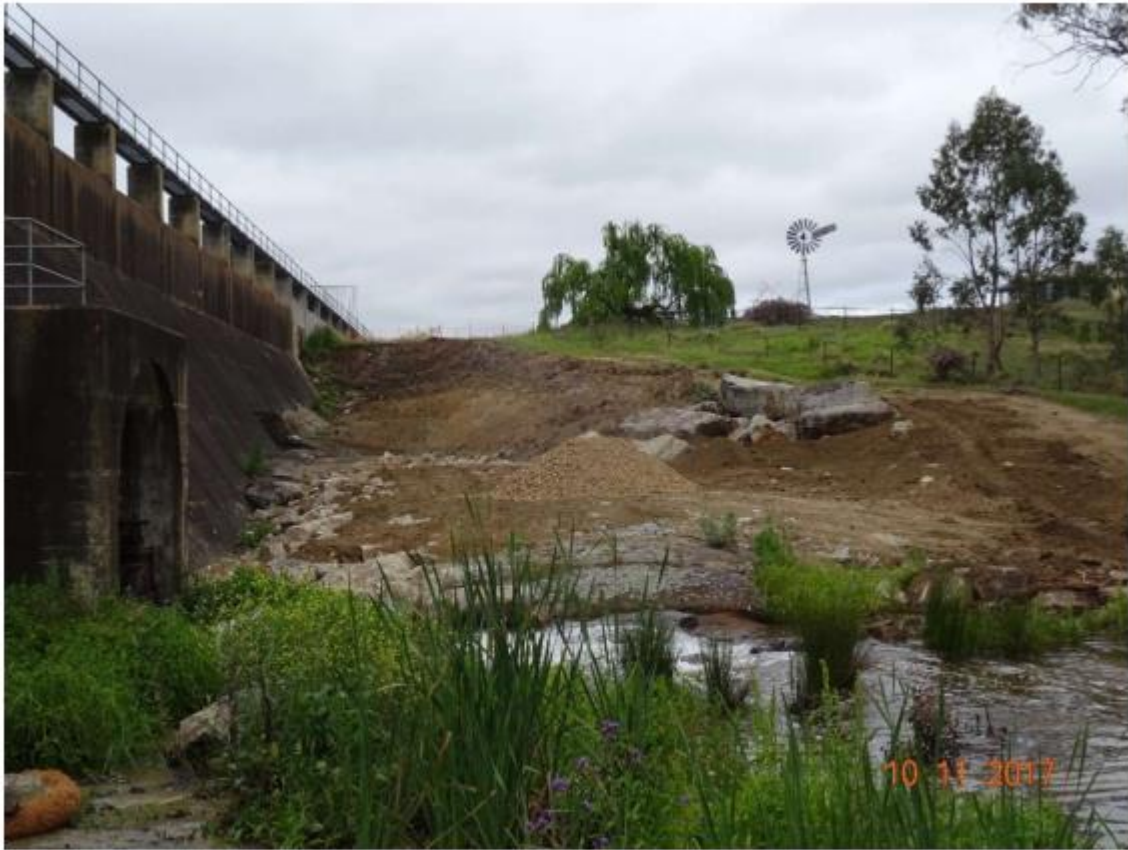
Excavation on LH Abutment
