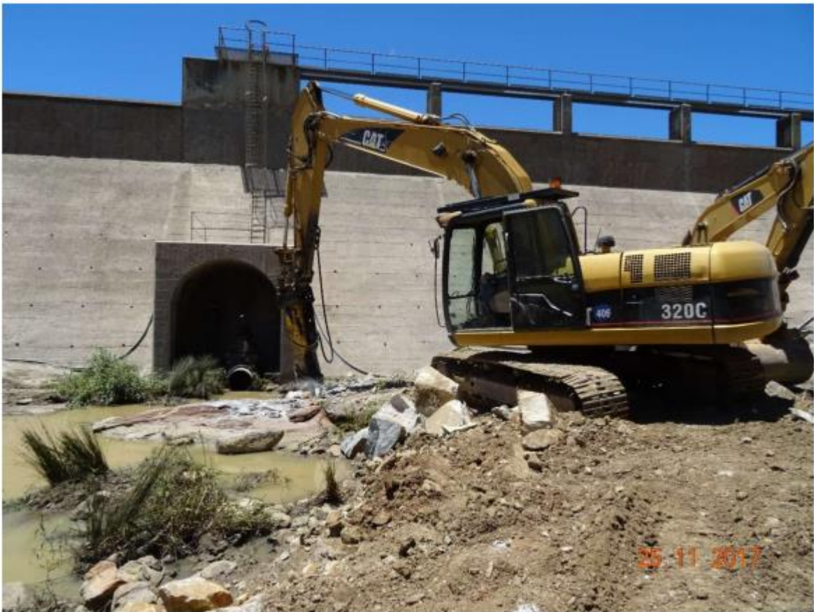
Excavation of Valve House Extension
