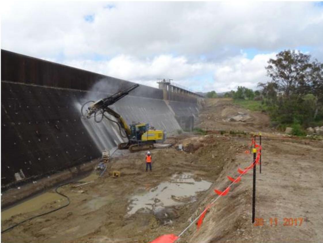
Drilling Anchors RH Abutment
