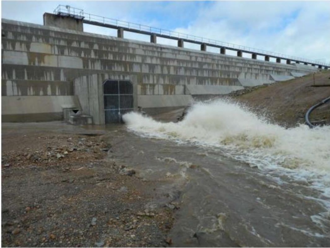
Testing of the Scour Valve System
