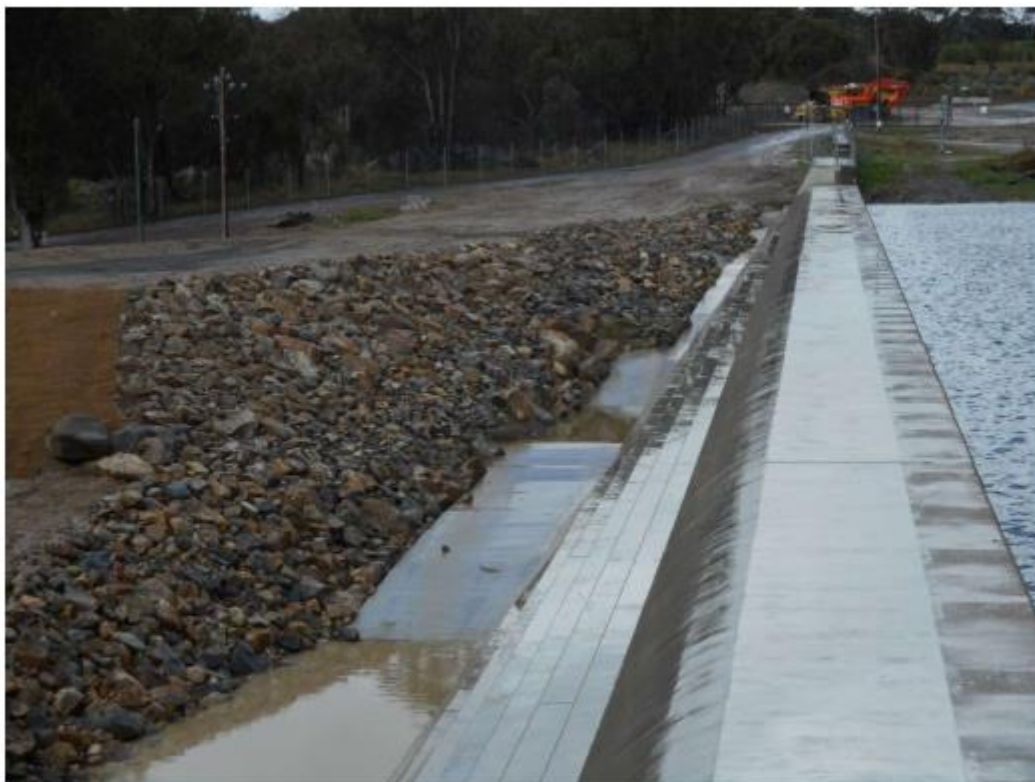
Photo Showing Completed RH Abutment, Bladder Pond and Rock Protection
