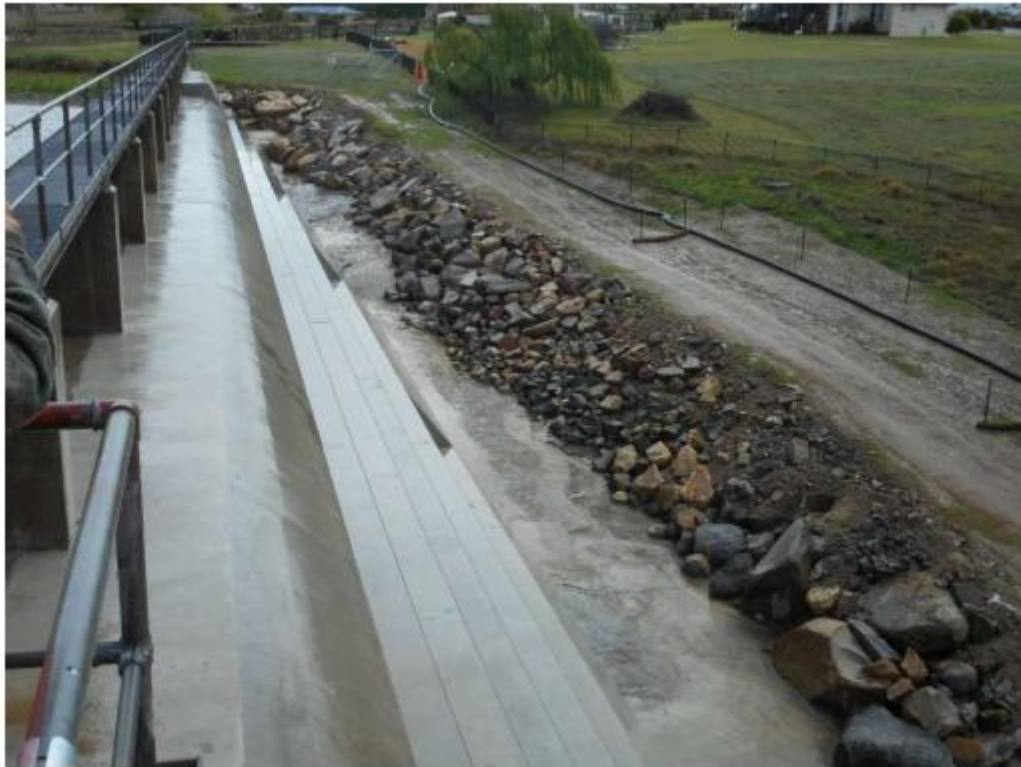
Photo Showing Completed LH Abutment with Rock Protection
