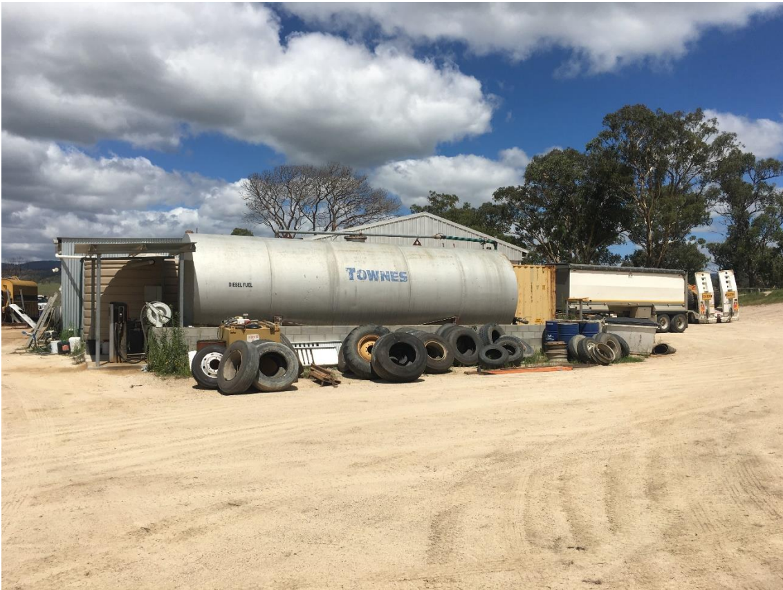
Photo: Bunded Diesel Fuel Tank
