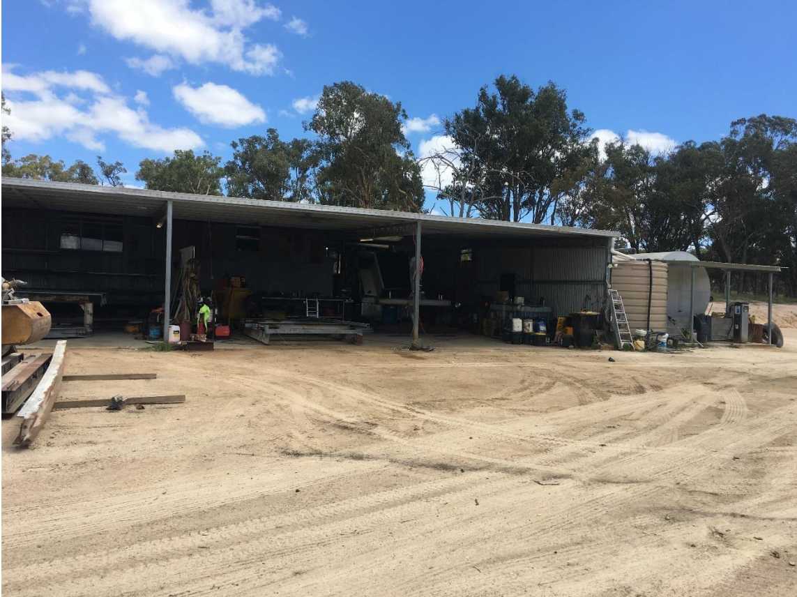
Photo: Northern Side of Workshop
