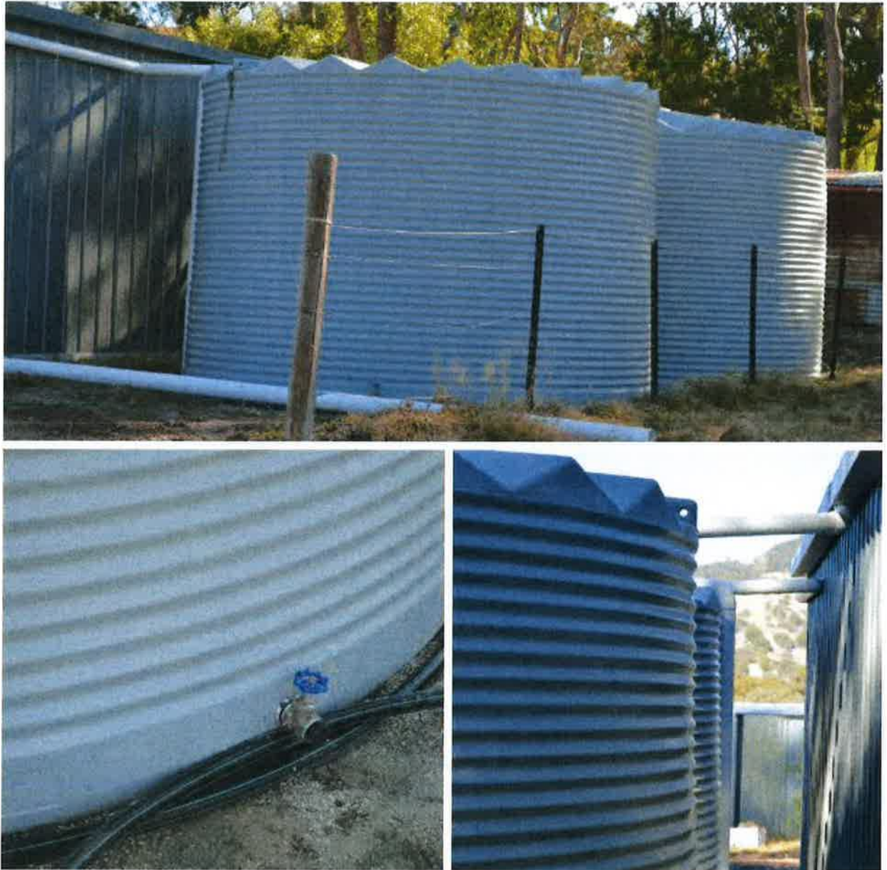
Figure 2 – Water Tanks, located adjacent to the recently installed shed
