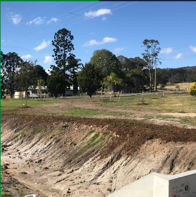
Improvements to public spaces
