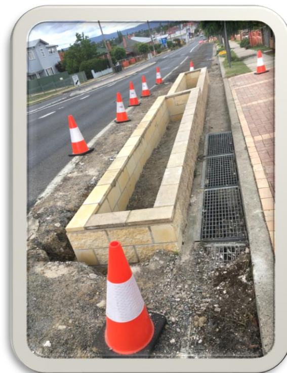
Figure 2, 3 and 4 New main installation and garden bed re-instatement narrowing to ensure worker safety
