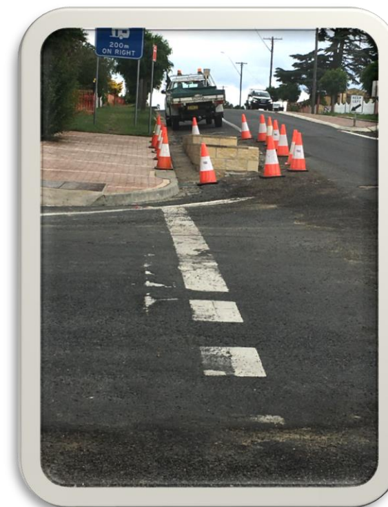
Figure 2, 3 and 4 New main installation and garden bed re-instatement narrowing to ensure worker safety
