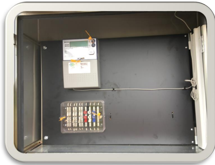
Figure 1 Completed meter installation RFS January 2021
