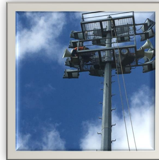
Figure 3, 4 and 5 New hardware for Flood warning system, new sirens and installation on the Federation Park light tower
