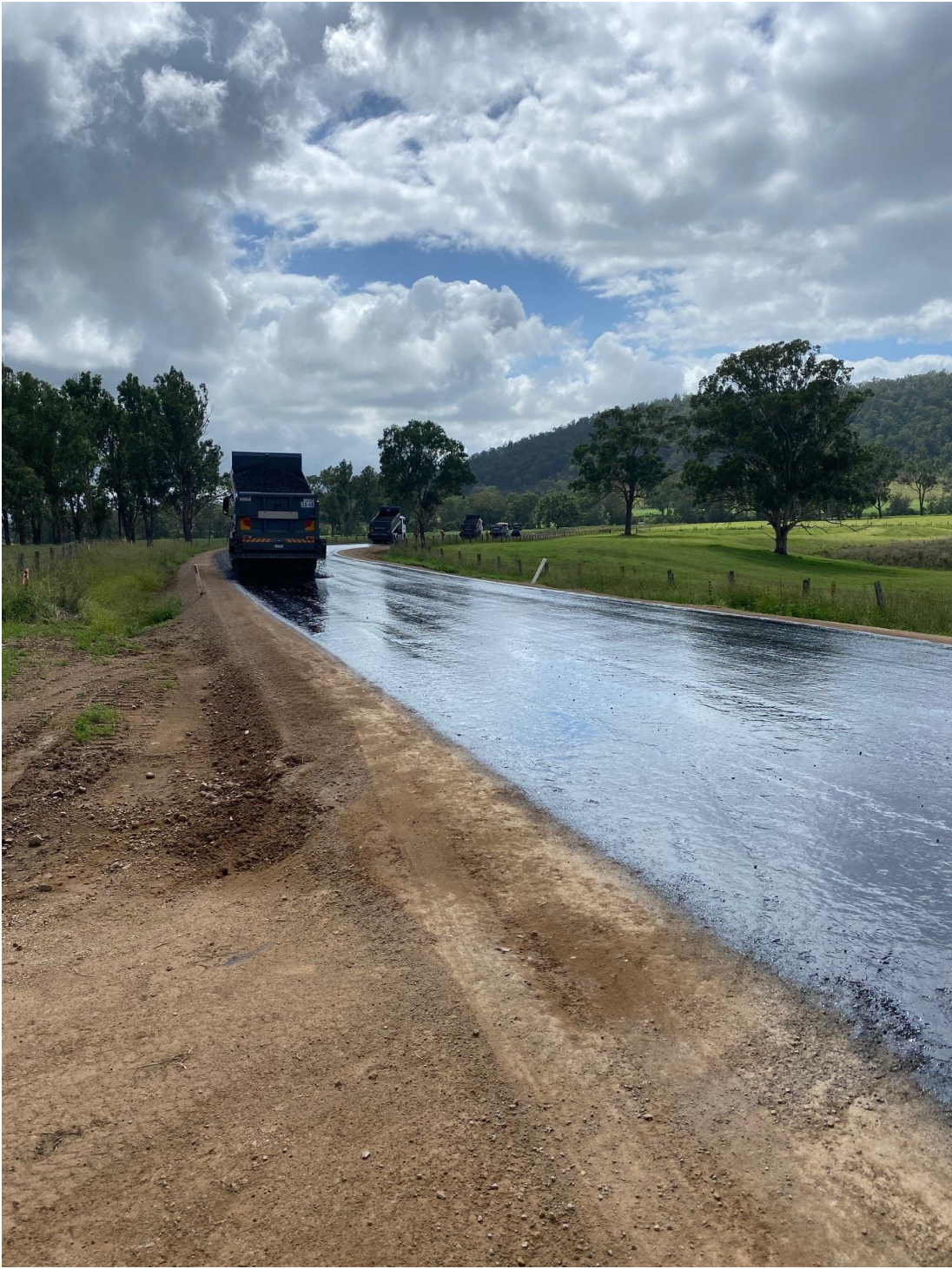
Sealing Works – Tooloom Road
