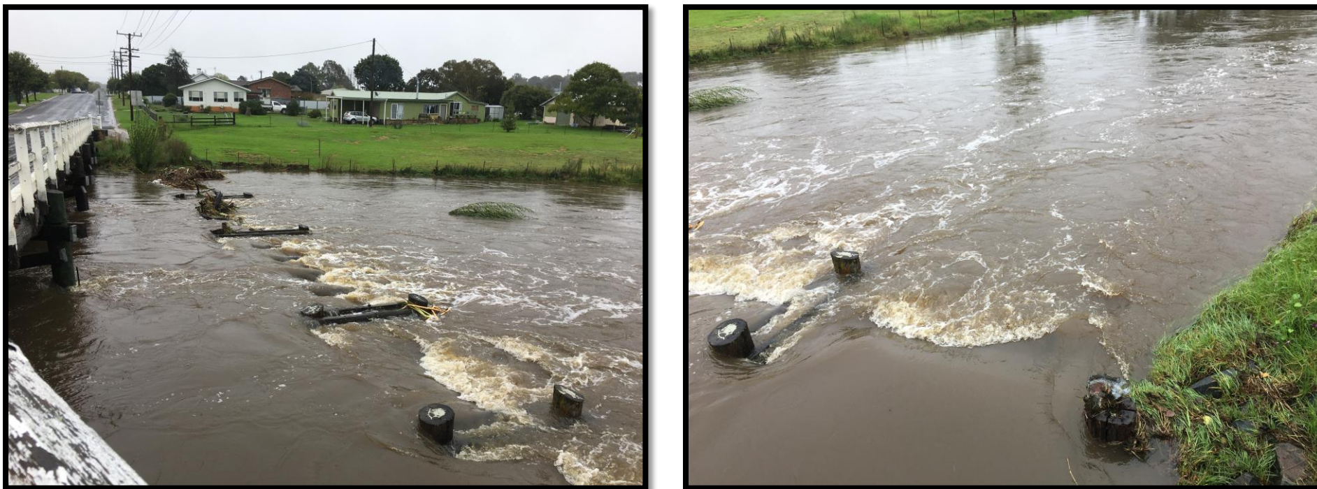
Figure 1 and 2 Flooding and Debris on the Molesworth Street Sewer Aquifer
