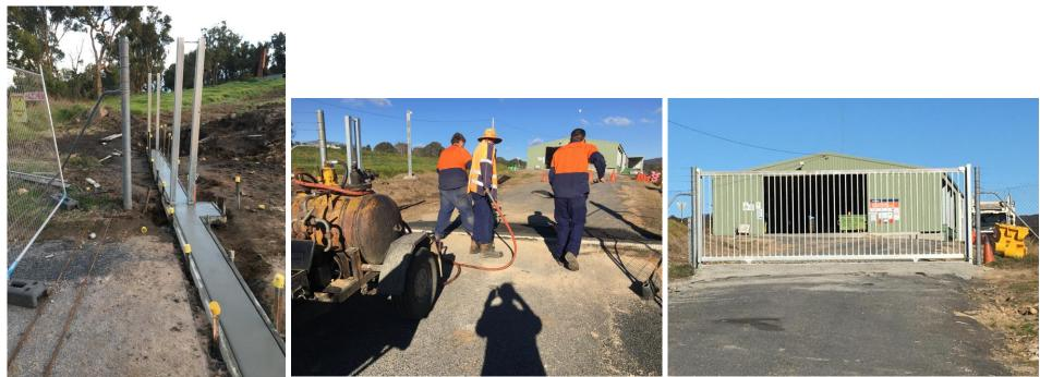
Figure 13, 14 & 15 Installation of concrete footings for gate track, Re-bitumen of surface and Gate installed
