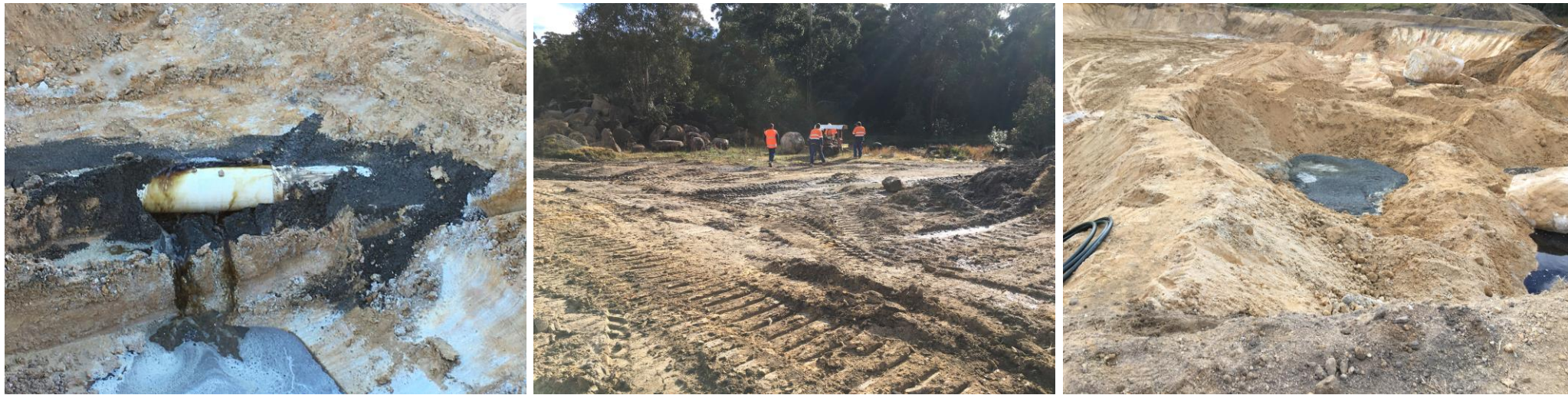
Figure 8, 9 & 10 Exposed leaking pipe, Water and Sewer crew and repaired encased pipe.
