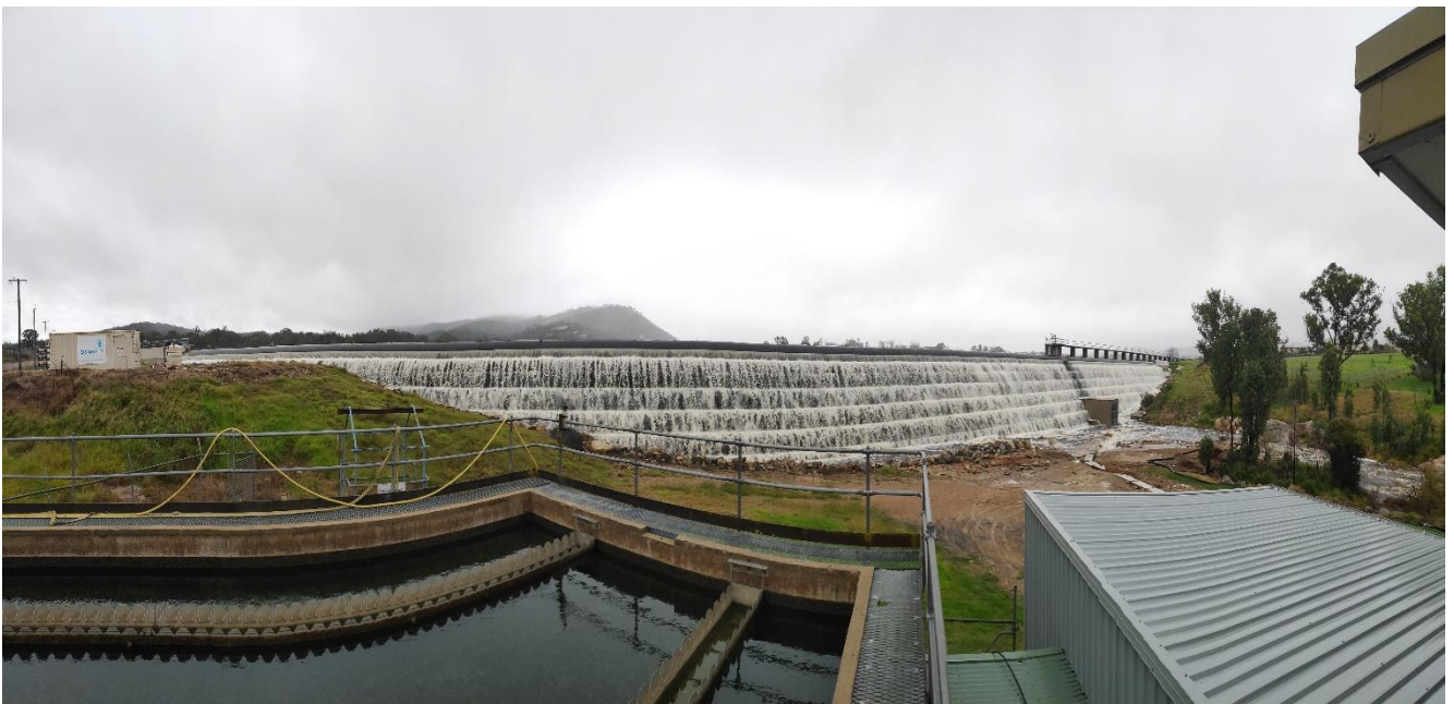
Figure 1: View of Dam Wall 9 April 2021
