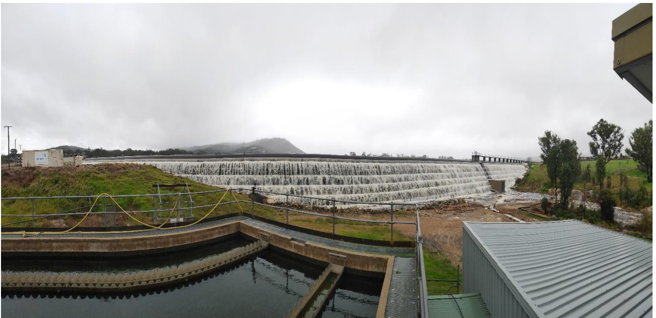
Figure 1: View of Dam Wall 9 April 2021
