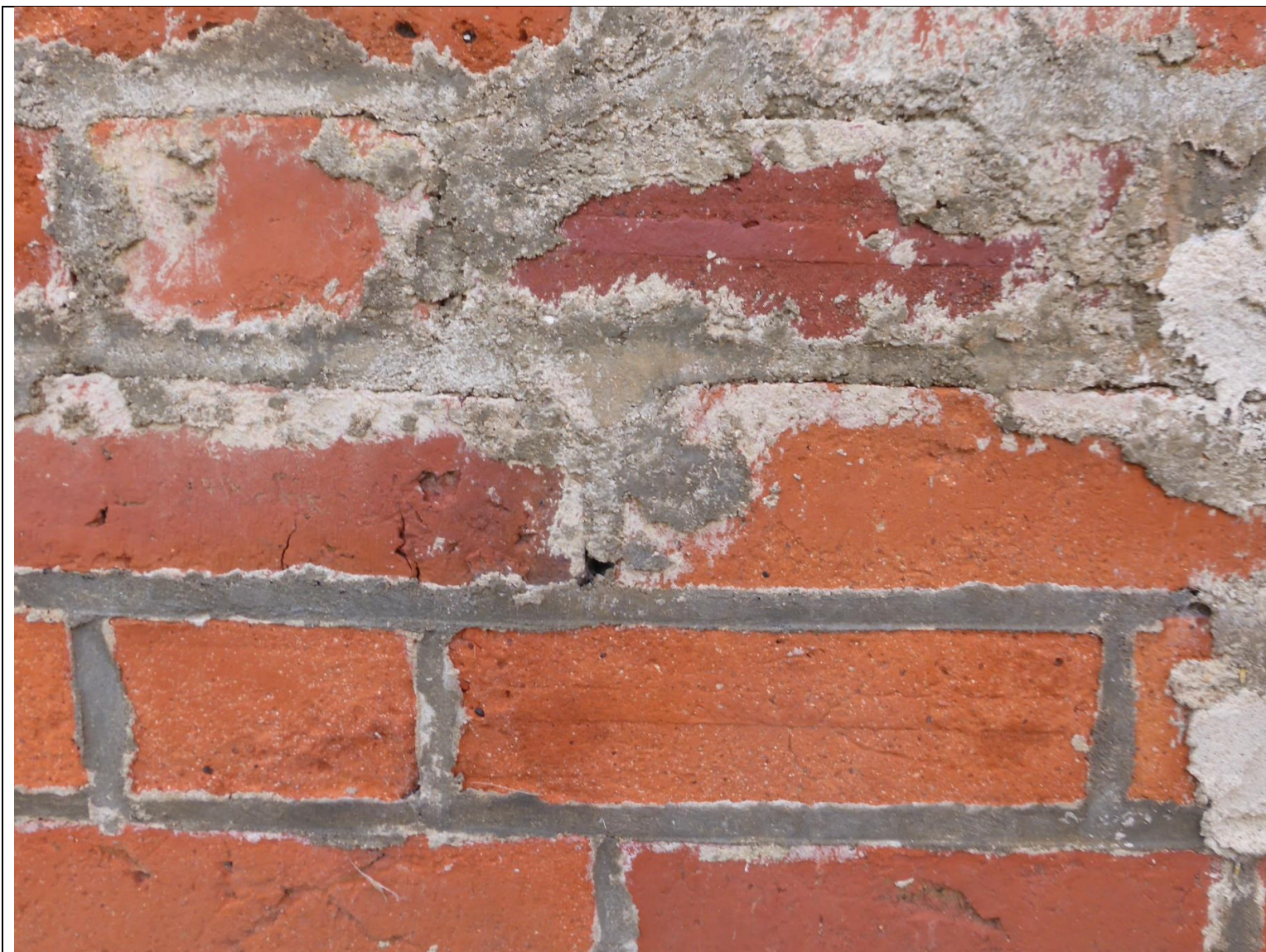
Previous inappropriate hard cement mortar repairs
