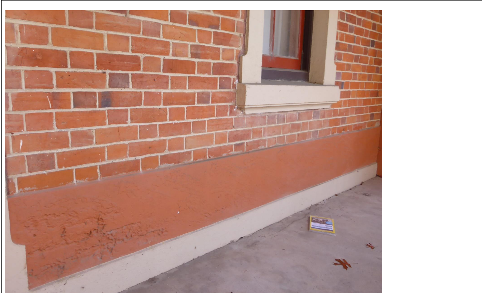
Existing concrete plinth under verandah cover on eastern wall. Note salt deposits / efflorescence on brick under window.
