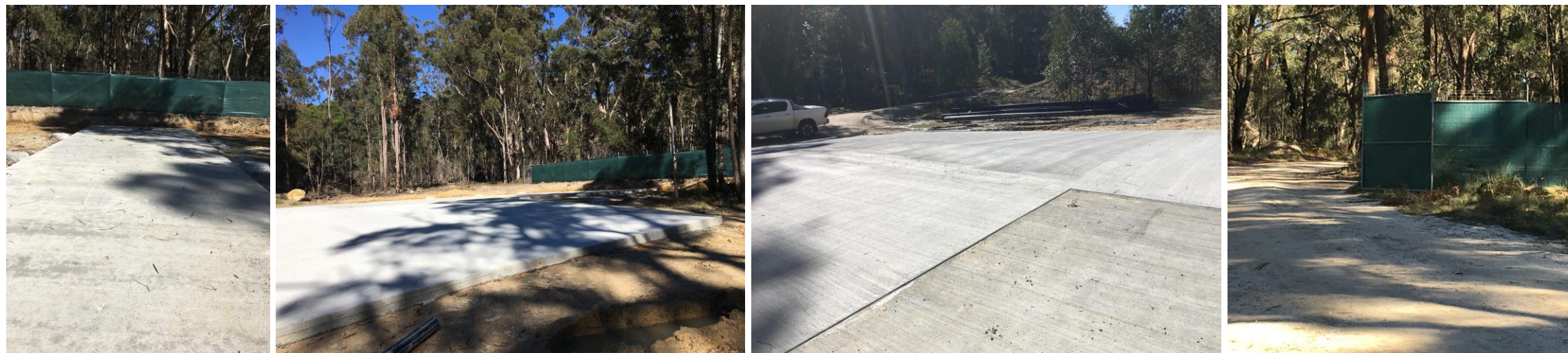
Figure 5, 6, 7 & 8 Slab completed & litter prevention fencing at Boonoo Boonoo August
