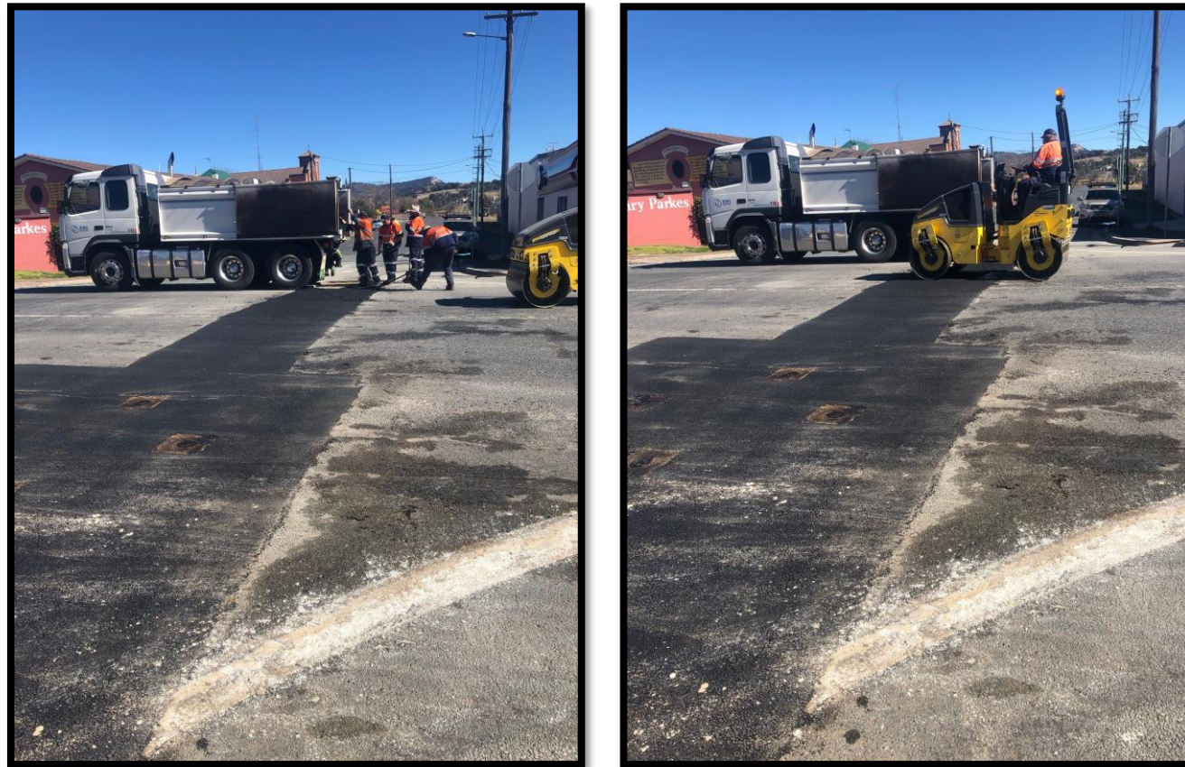
Figure 1 & 2 Installation of asphalt on the New England Highway
