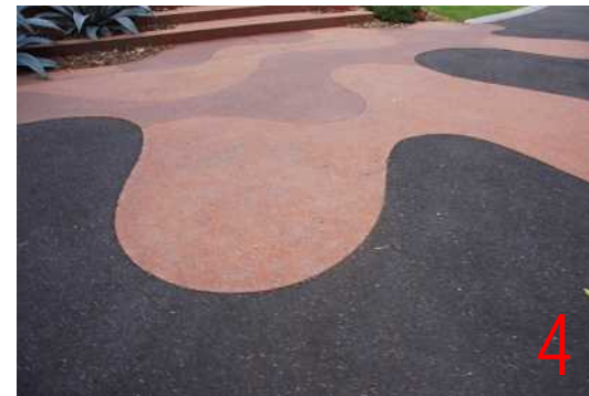
Exposed concrete paving
