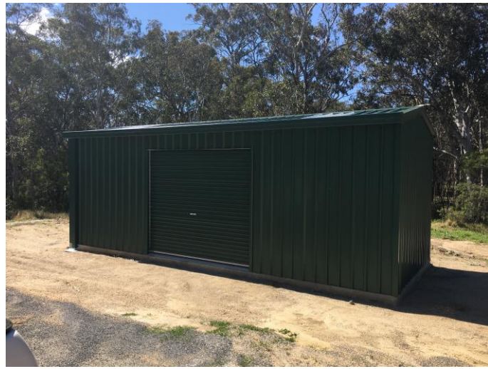
Figure 1 Liston Tip-shop completed September 2021
