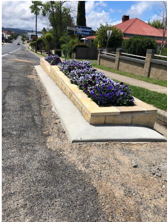
Figure 1 Installation of garden bed curbing on the New England Highway
