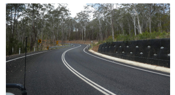
495 km sealed roads
