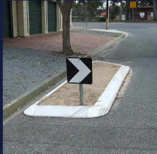
Installation of Traffic Calming Kerb Blisters
